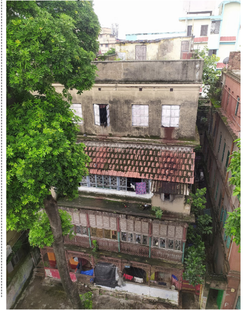
Example of using Same Repair material & Technique Case of settled Kori-Borga roof repaired by rebuilding the entire bay using same material and technique
